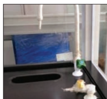
Drip cup, water faucet type and location
