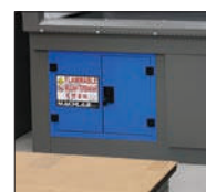
Flammable/corrosive chemical safety cabinet
