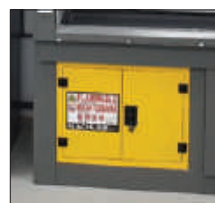
Flammable/corrosive chemical safety cabinet
